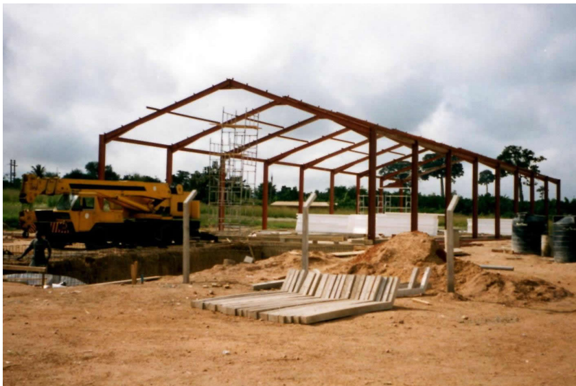
Above: Our first factory being constructed in Ghana.
